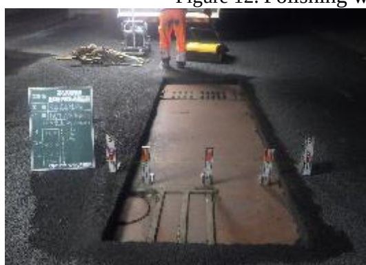
Figure 13. Repair work for steel bridge slab using new material.
