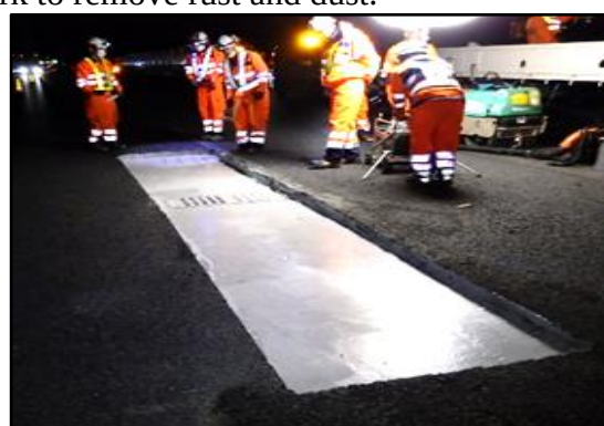
Figure 13. Repair work for steel bridge slab using new material.
