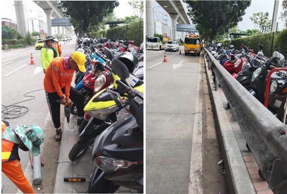
Figure 3 Install guardrail along the roadside to make longitudinal boundary.
