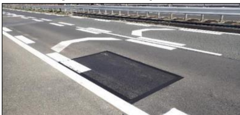
Figure 11. Appearance 60 days after repair work
