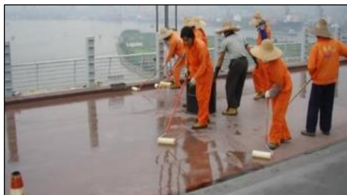
Figure 6. Steel bridge slab adhesive using epoxy-based material in China
