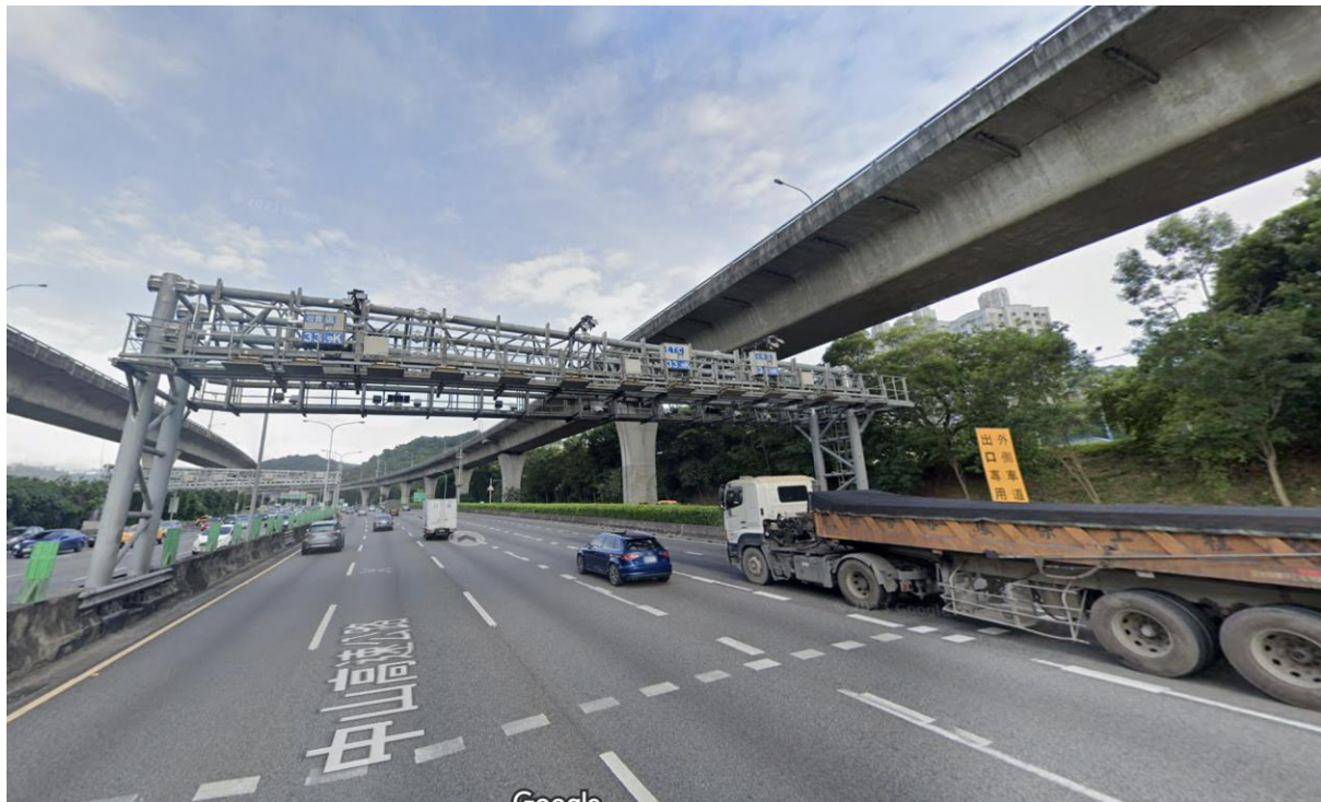
Figure 2 ETC Gantry
